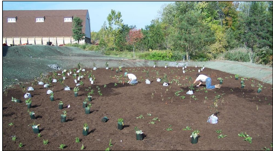
Figures 4.55 - 4.56. The Town of Penfield has a rain garden located along Jackson Road that provides a good example of how to sustainably address stormwater runoff. These images show a new planting (top) and the same garden after several years (bottom).
