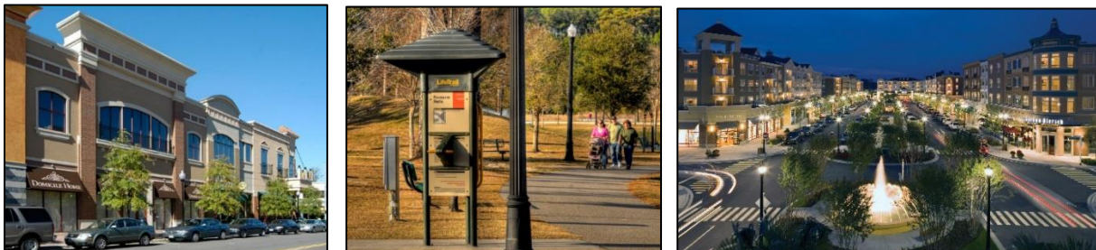
Figures C.18 - C.20. The Market Common transformed a former air force base into a mixed-use development.
